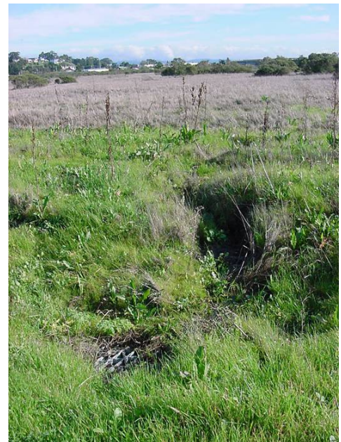
Fig.B.9 Drain Inlet for Basin 3
