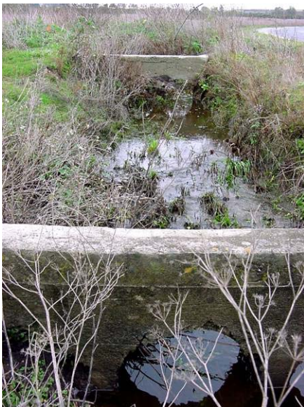
Fig. B.6 Concrete headwalls in drainage
