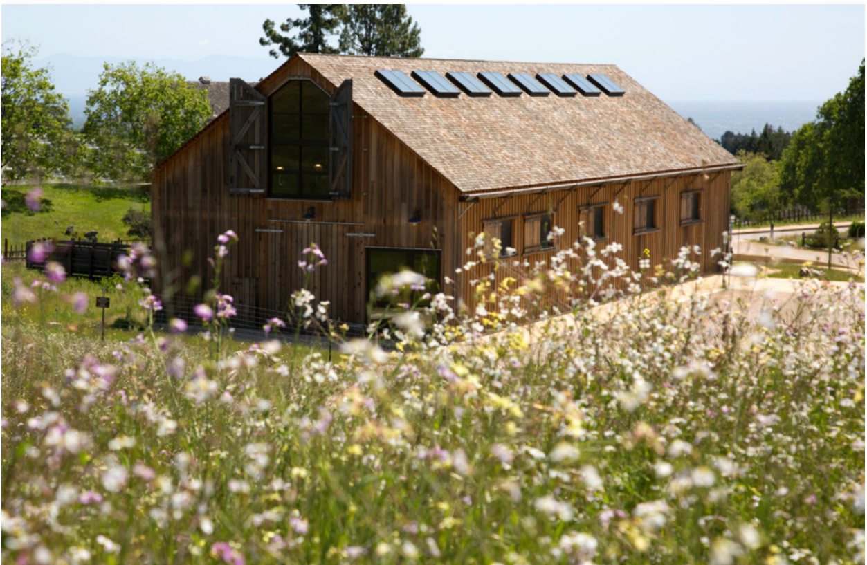
▲ Renovated Hay Barn
